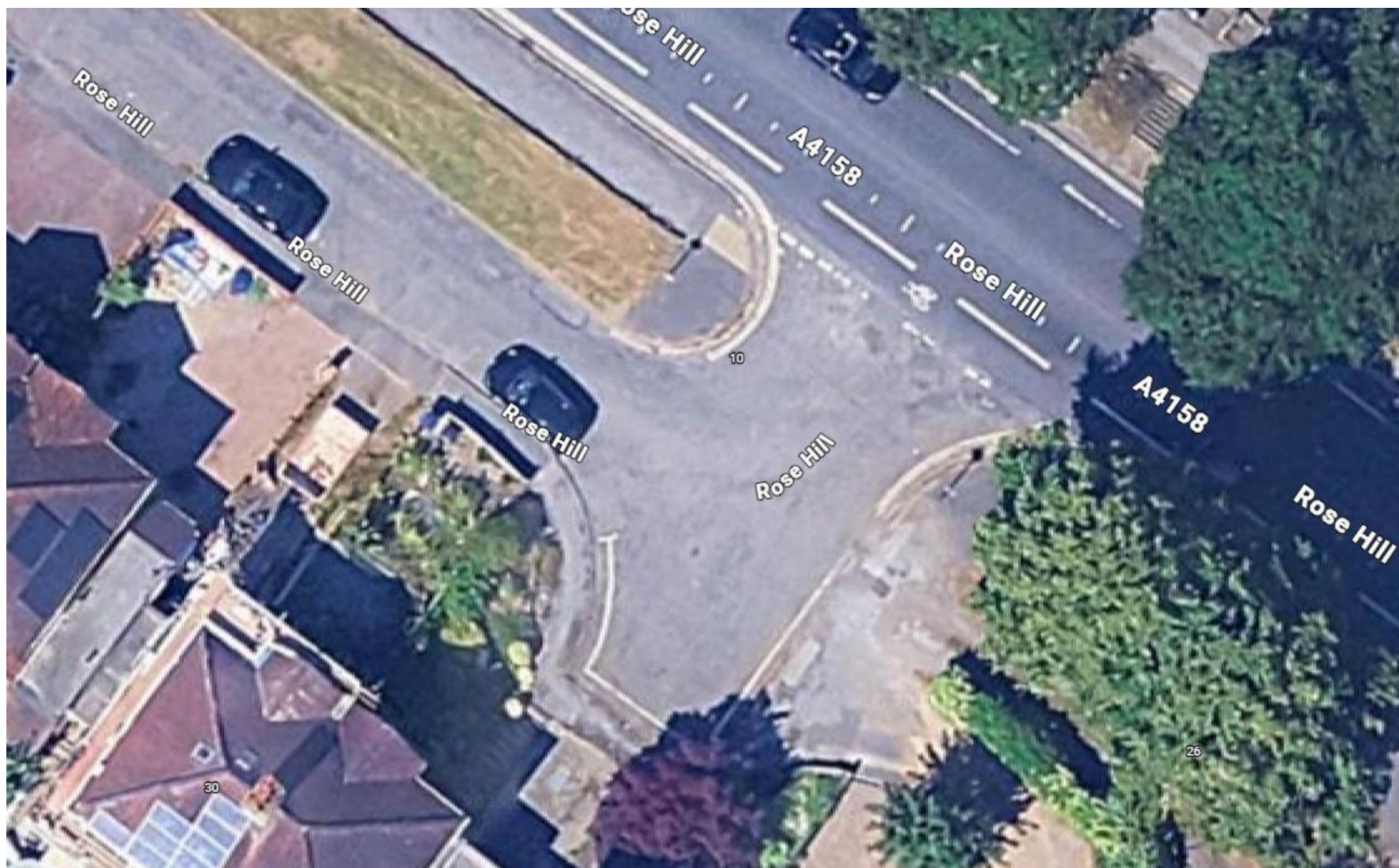
Service road southern access
